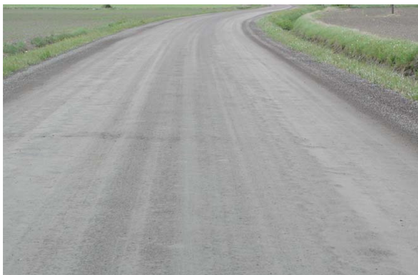
Figure 2: Surface condition of firm and well performed test road in July 2001
