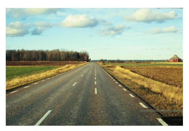
Figure B.2 - Broken line: 3 + 3 m; width: 10 cm
