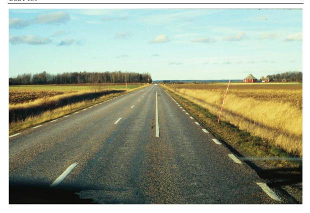
Figure B.3 - Continuous line; width: 10 cm
