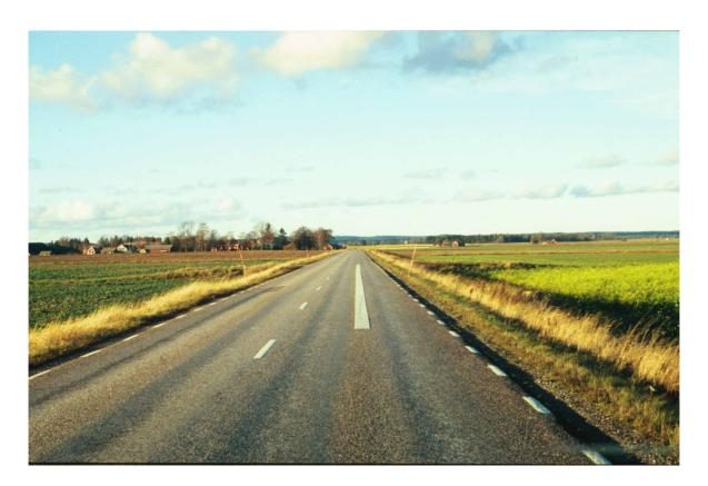
Figure B.4 - Continuous line; width: 30 cm
