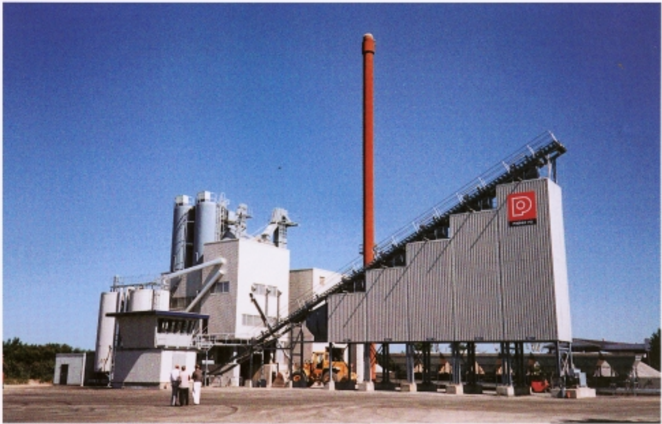
New asphalt plants are enclosed to minimise noise and dust problems.
