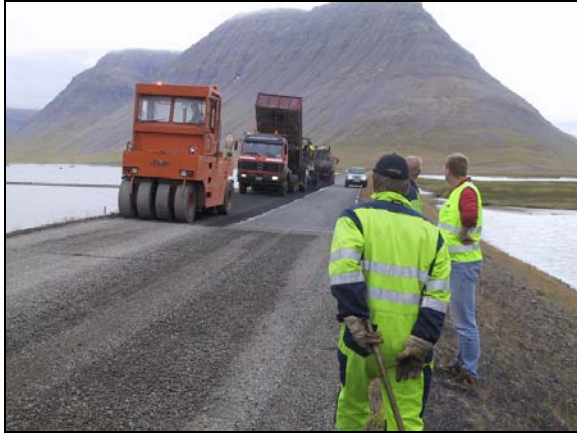
Figure 2 Laying of Vadall section
