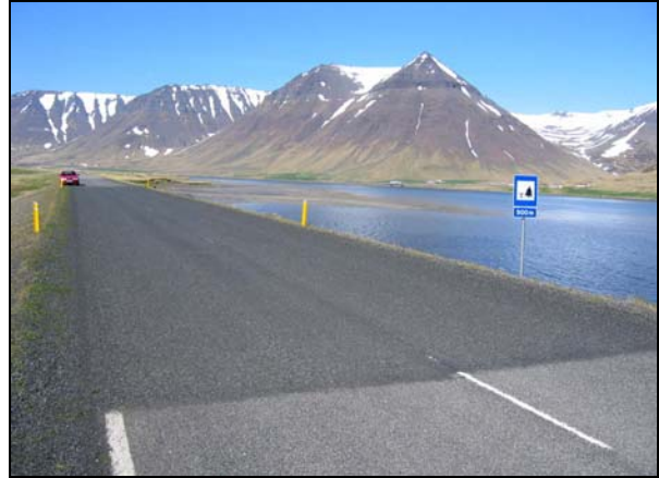
Figure3 Overview at Vadall section
