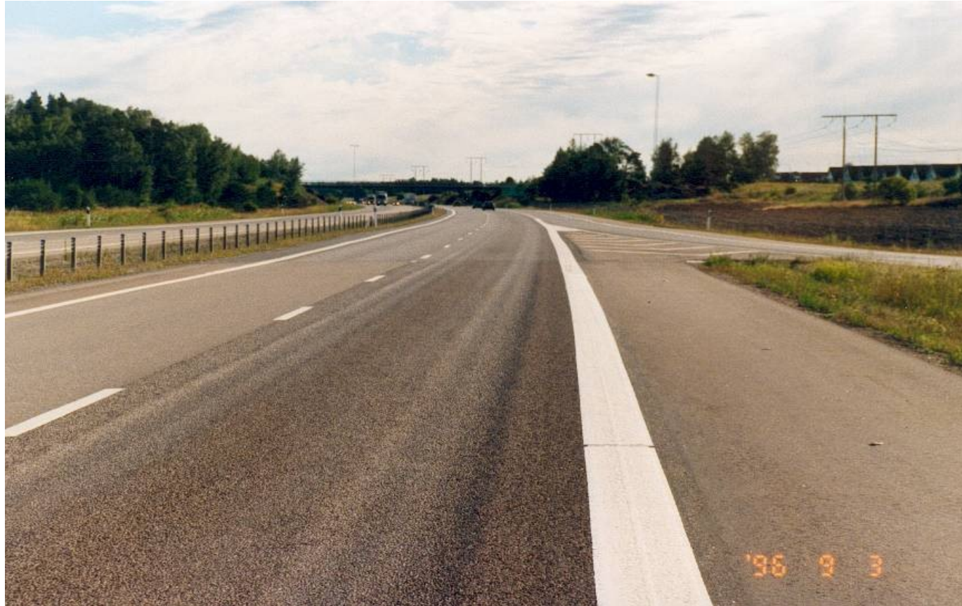
Rutting caused by heavy trafik
