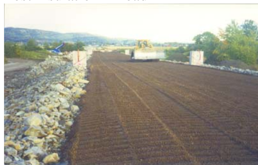
Frost insulation in road
