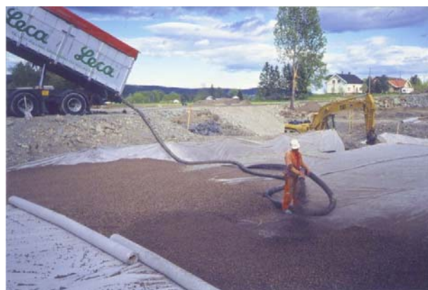
Frost insulation in road
