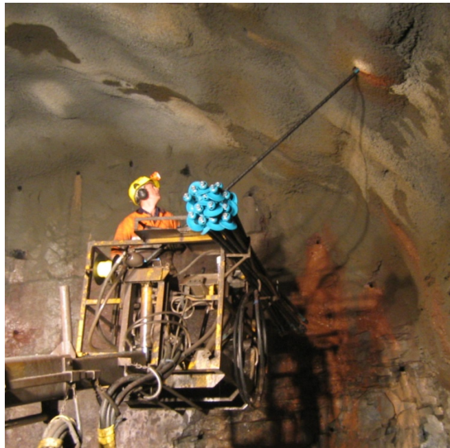
Figure 4-8: Installation of rock bolts in Fáskrúðsfjörður tunnel [46].
