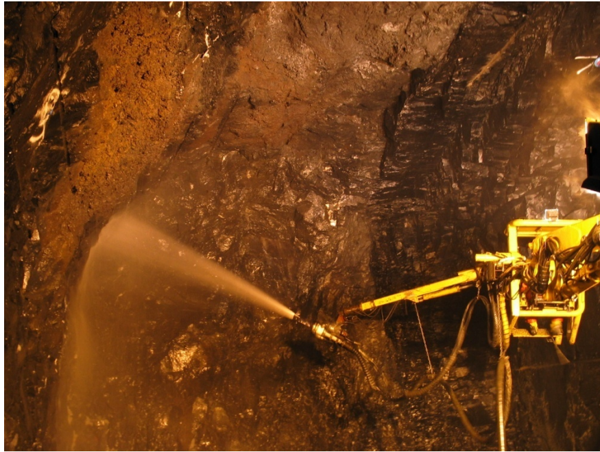
Figure 4-11: Shotcrete applied on a wall in Fáskrúðsfjörður tunnel [46].
