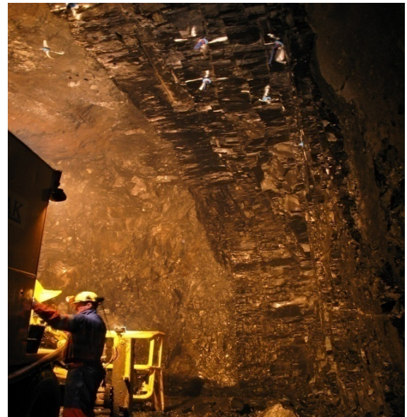
Figure 3-13: A dike in Fáskrúðsfjörður tunnel [46].
