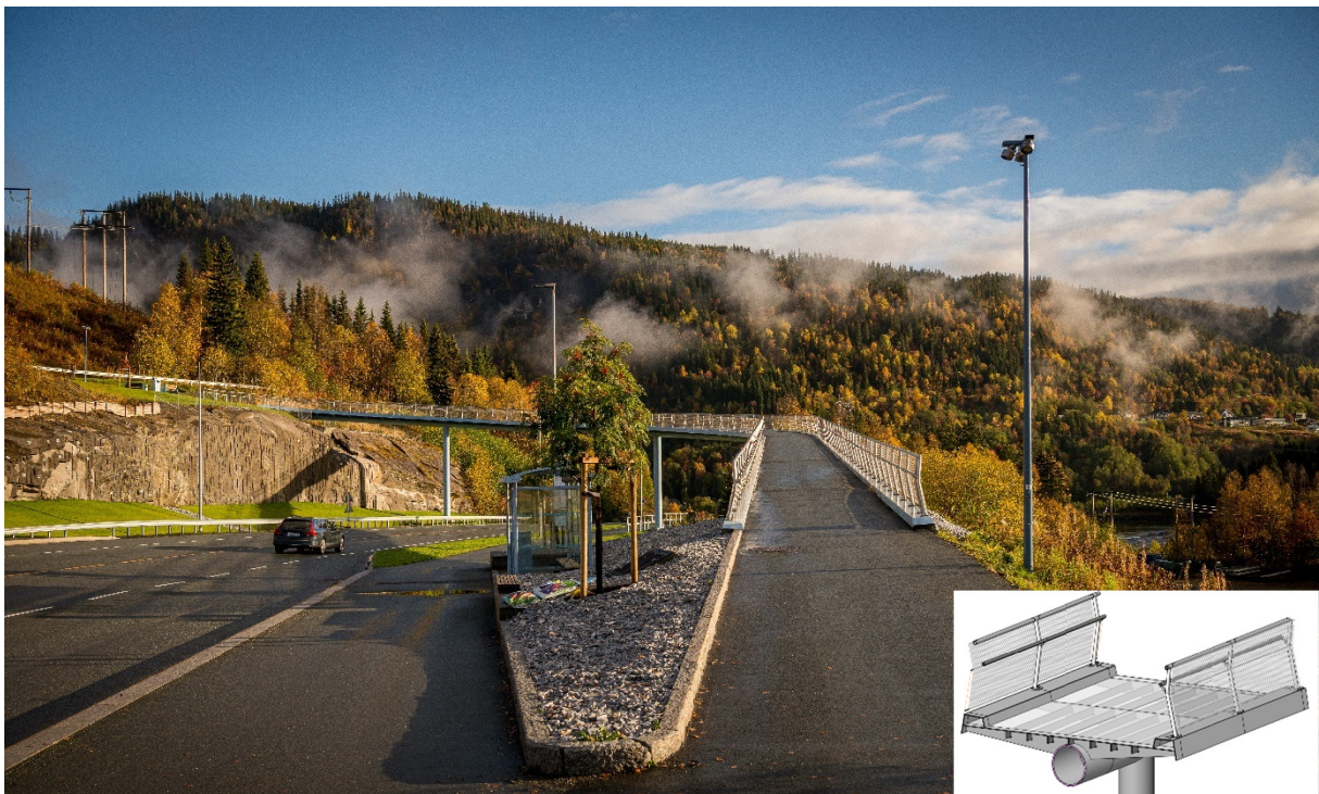
FIGURE 11: Mjølan footbridge as built
