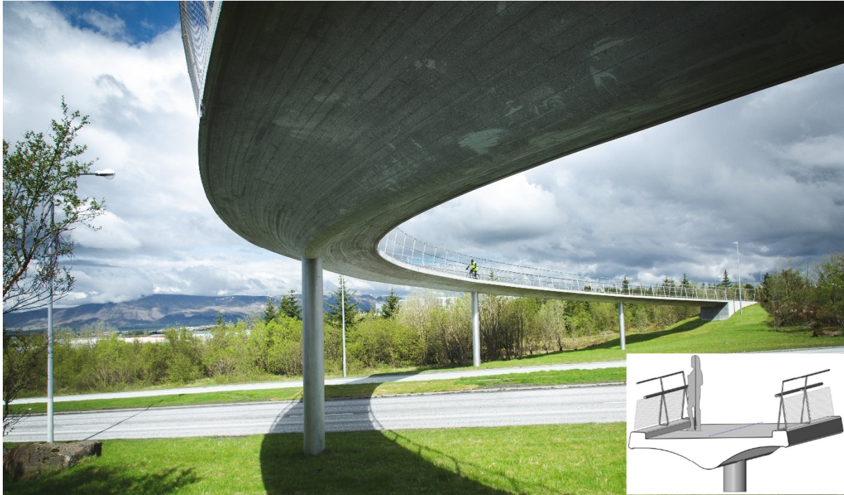
FIGURE 12: Breiðholtsbraut footbridge, a reference in comparison to a steel girder in the Mjølan footbridge pre-design
